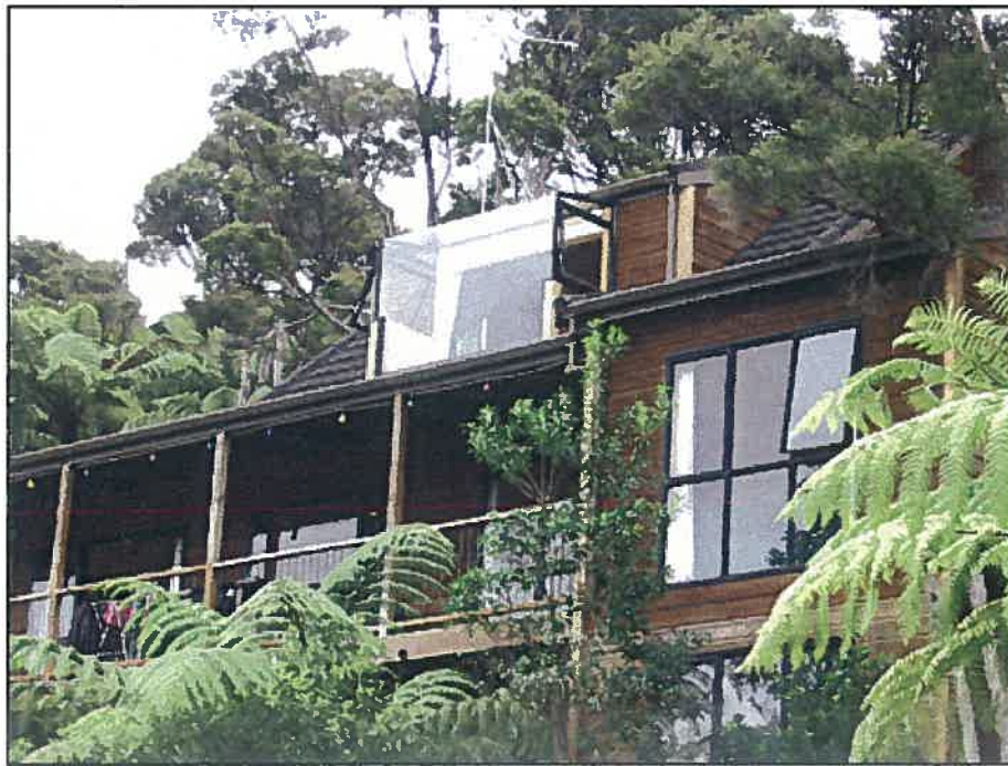
View of upper floor looking South West.
