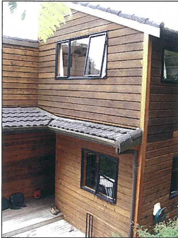
View of right-hand side elevation looking South East.
