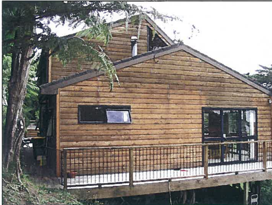
View of left-hand side elevation looking North East.
