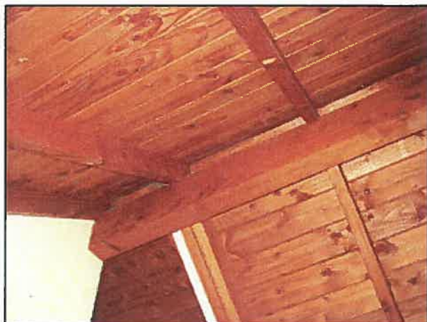
Internal views of rear roof plane framing.
