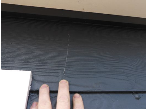
Cracked cladding
