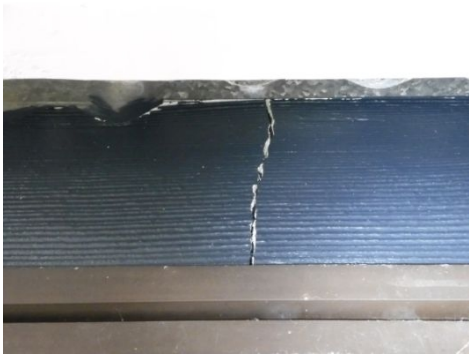
Cracked cladding
