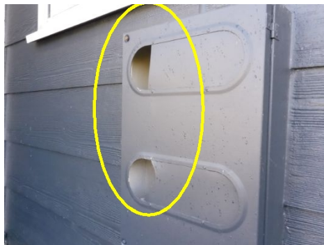
Damaged perspex
