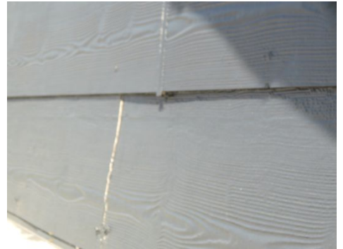
Cracked cladding
