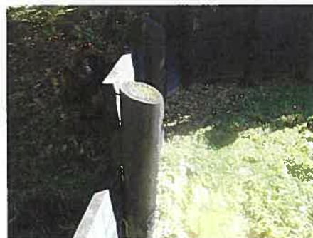
Some damage present
