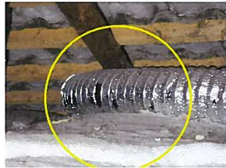
Damaged ducting
