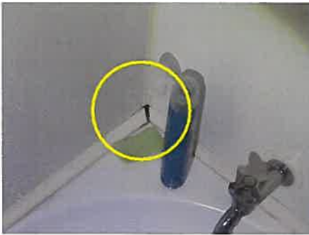
Poorly sealed
