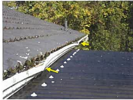
Damaged guttering
